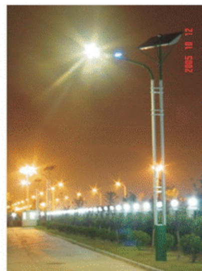
Wuxi new area road lighting project
