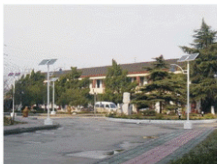
Wuxi city police station college lighting project
