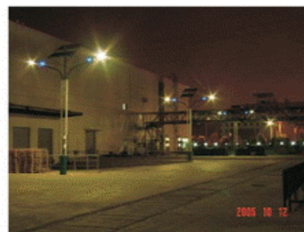
Wuxi shangde company factory lighting project
