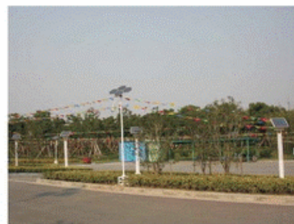
Wuxi city lihu park lighting project
