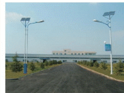
Zhenzhou development zone factory lighting project
